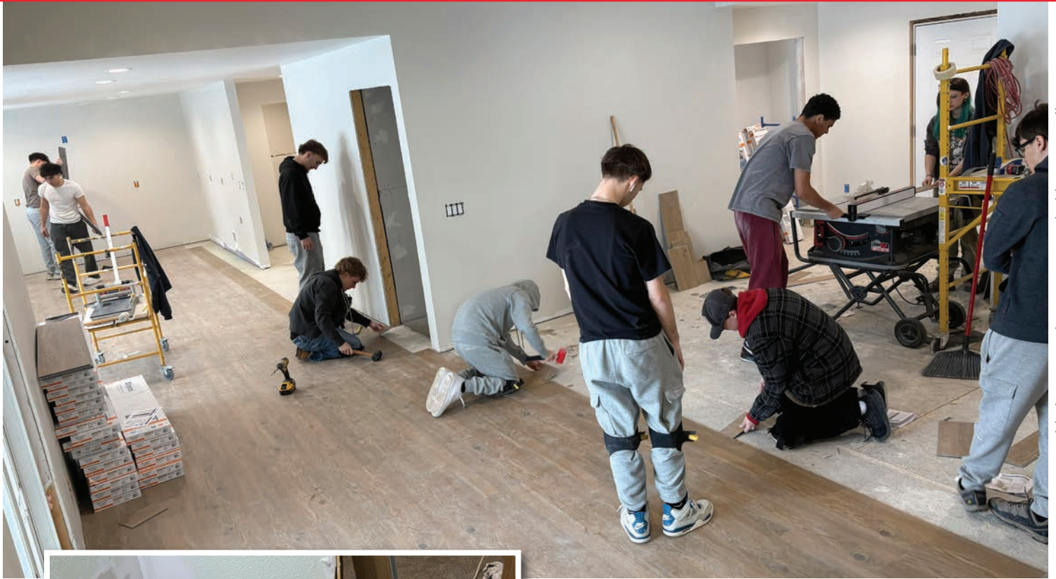
Trojan Build photos on this page provided by Tom Bell
