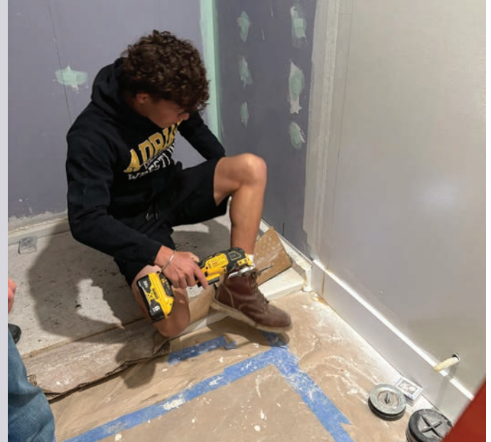
Trojan Build photos on this page provided by Tom Bell
