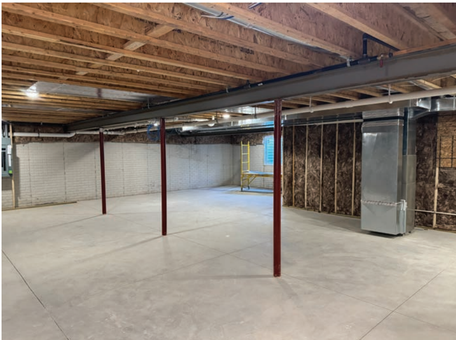
The full, unfinished basement offers plenty of room for storage or the potential to finish and customize for the buyer's needs.
